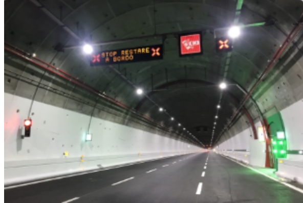
DBA – SANTA MARIA AND BOSCACCIO TUNNELS
